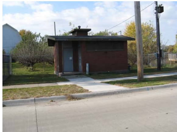
Bond Street Lift Station
