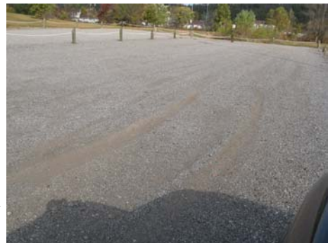
Parking Lot Surfacing
