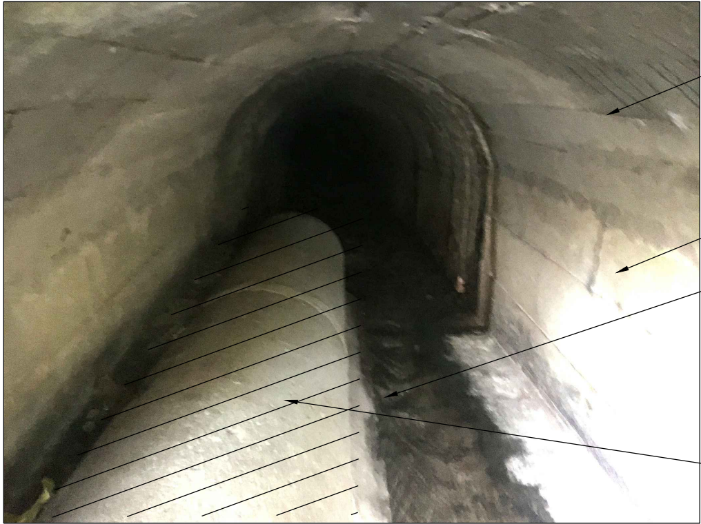
PHOTO 3: INTERIOR OF UWBS SHOWING EXISTING COMBINED SEWER PIPE
