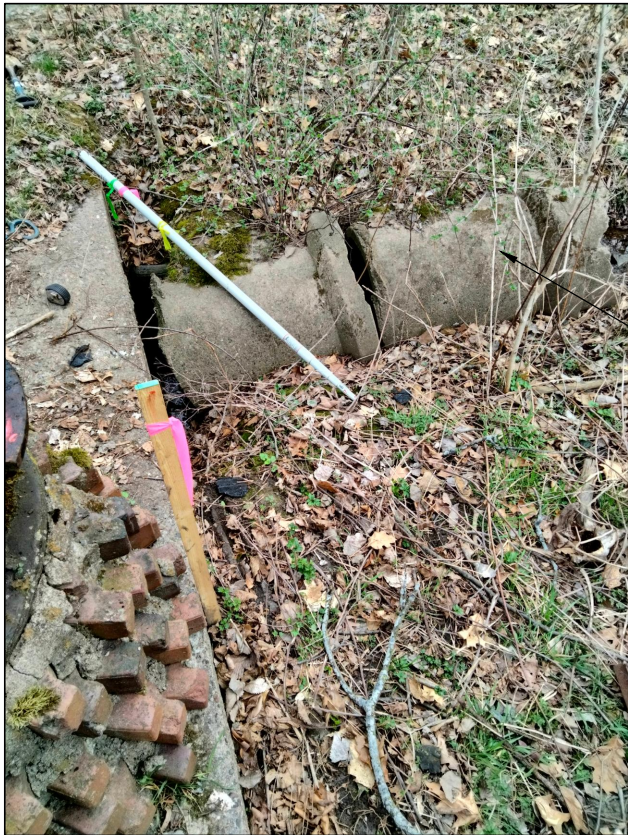
PHOTO 1: UWBS BROKEN PIPE SOUTHEAST OF UWBS
