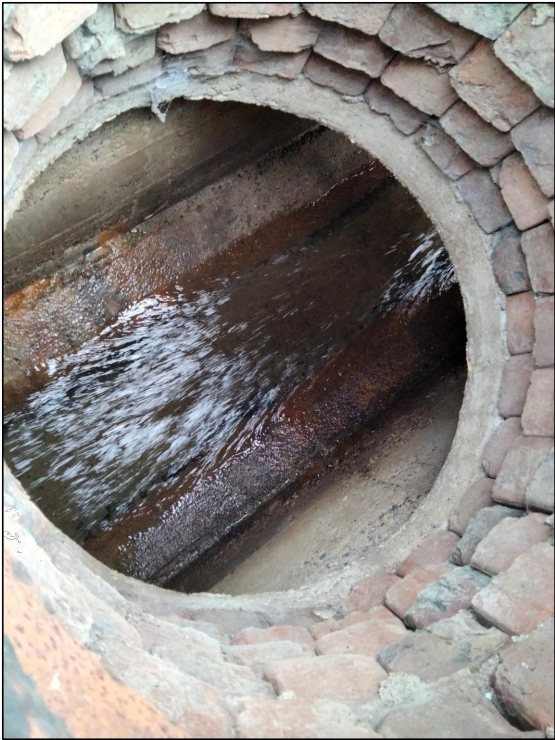
PHOTO 3: MANHOLE 5455 - APPROXIMATELY 5 LAYERS OF BRICK RISER
