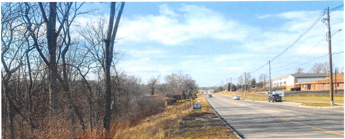
On Colorado Street looking west along the north property line towards Heartherlyn Drive
