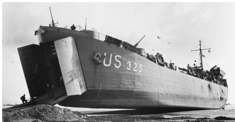
These ships could carry 20 Sherman tanks in the giant hold within the ship. They were the only ships ever made that could go anywhere in the world and deposit their cargo onto a hostile
