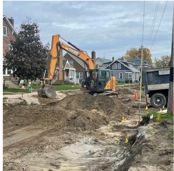
Dirt removal and leveling of the street surface are part of the preparation for paving on Sycamore Street that was accomplished Tuesday (Oct. 24). Work will continue to prep the first two blocks for paving as weather permits.
