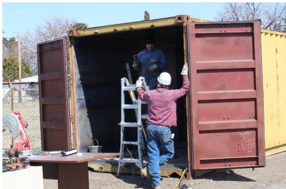
to be built to certain specifications and is lined with steel on the sides, the top, and on the bottom to absorb the heat of the fire. Behind that will be the control room where the instructors will maintain the fires.
