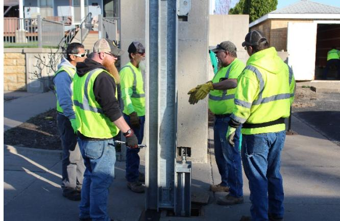
Exercising the flood gate involves the installation of each piece of the structure, physical inspection of each piece and accomplishing repairs as needed, and dismantling and proper storage of each piece of the structure. Training was supervised by staff members who had participated in a previous installation.
