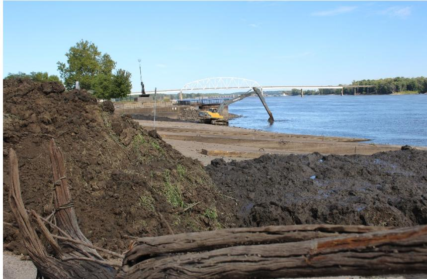
The piles of mud is scheduled to be hauled away next week depending on the length of time the dewatering process takes. Once the dredging operation has been completed and the piles of mud and debris are hauled away, the Muscatine Fire Department will clean the boat launch area by washing the remaining mud back into the Mississippi River.
