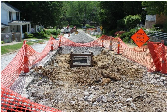
Underground work on West 8th Street and through the property at 891 West 8th Street continues as part Phase V of the West Hill Sanitary and Storm Sewer Separation Project. West 8th Street is currently closed to traffic from Climer to Lucas.
