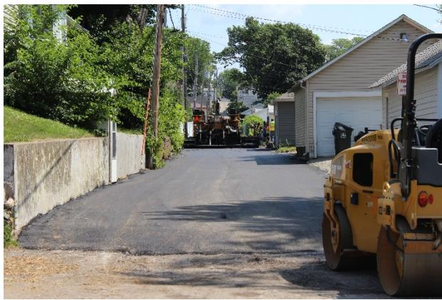
Paving of the nine alley and nine street segments, part of the 2020-2021 Street & Alley Asphalt Overlay Project, has been completed with Manatts returning in the next two weeks to wrap up the project with paint stripping and manhole adjustments.
