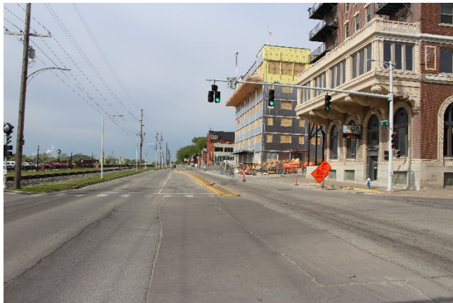
Mississippi Drive is pictured from Iowa Avenue toward Pine Street before the start of Phase I of the Mississippi Drive reconstruction project.
