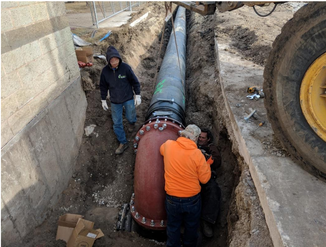
New pipe connection at WPCP head works January 26, 2018
