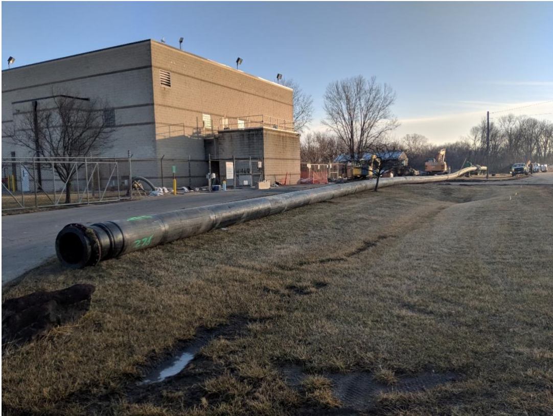
Fused pipe ready to be pulled into place at the WPCP January 24, 2018.
