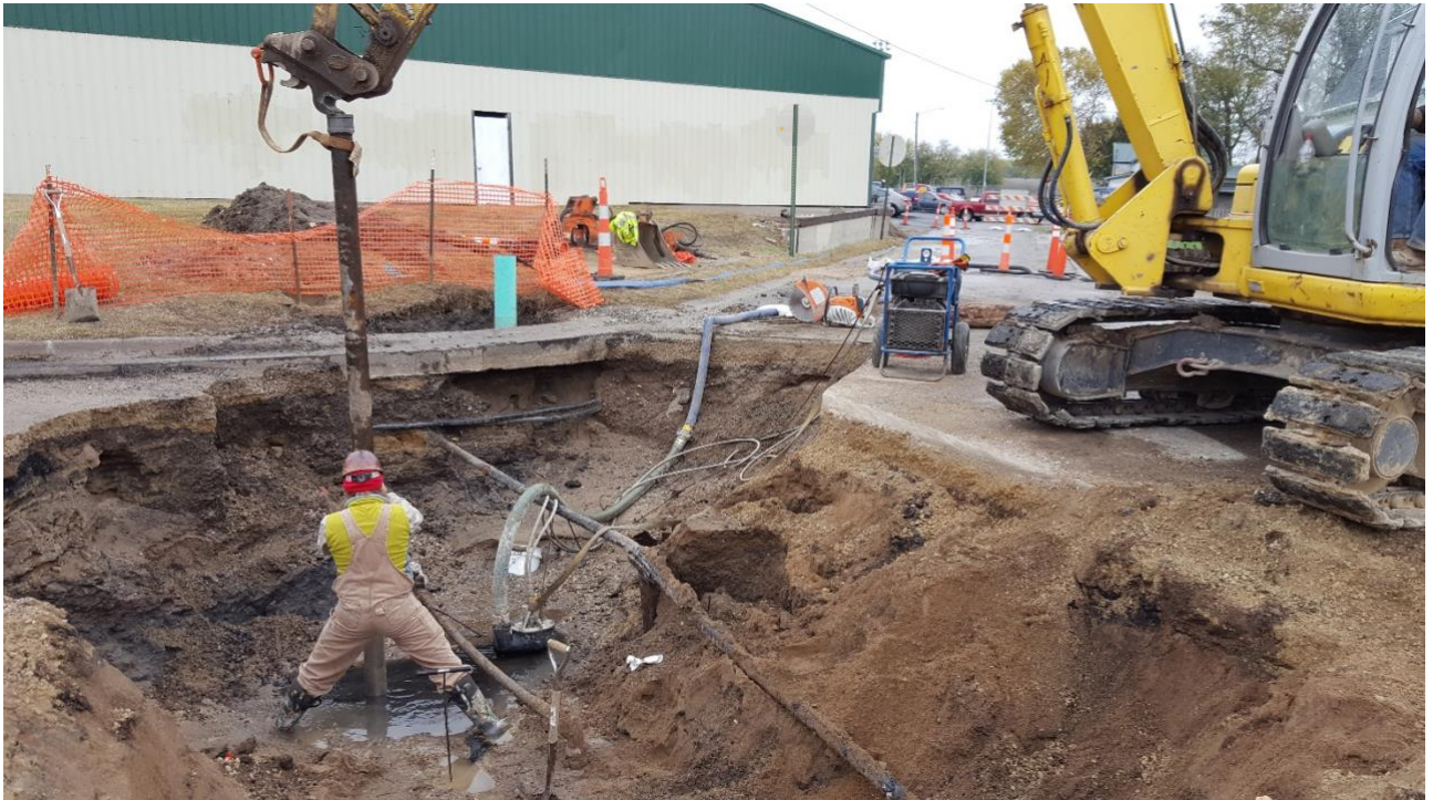
Discovery excavation to see where the leak was and if repair is possible October 31, 2017
