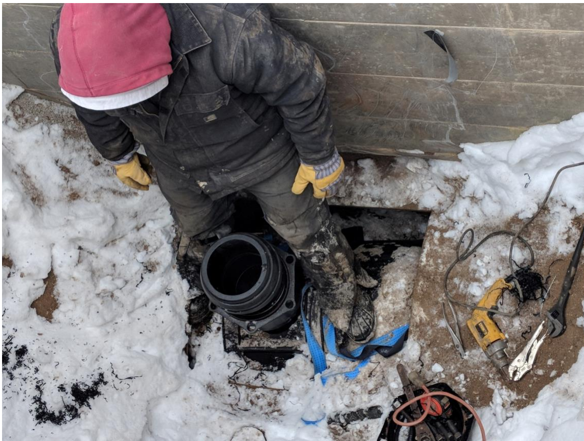
Schley lift station connection, cut in top of 30" exposing new 26" inside February 6, 2018
