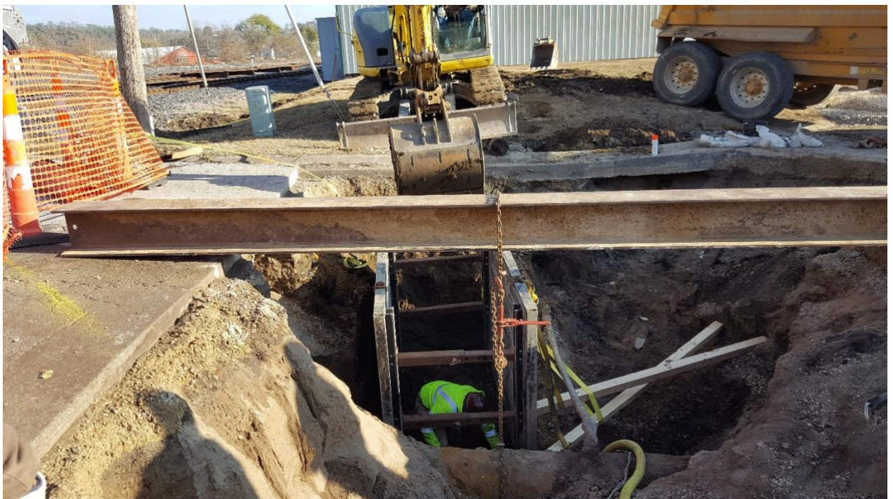
Chained 16" water main above sewer line leak, fear of damaging this pipe during any repair led to other options being considered. Water supplier could not guarantee isolation of this main. Small 2" connection coming off the top of the water main was very vulnerable. November 8, 2017.
