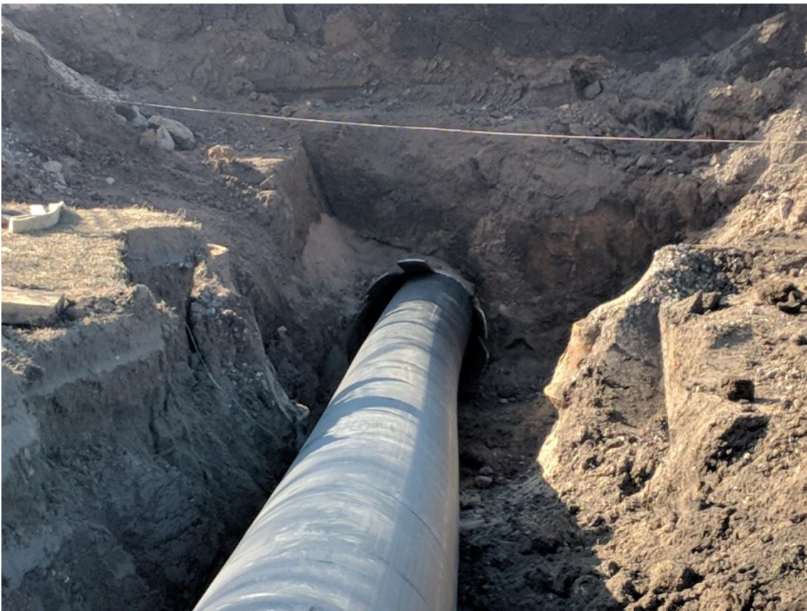
New pipe entering 30" at WPCP as it is being pulled through January 22, 2018
