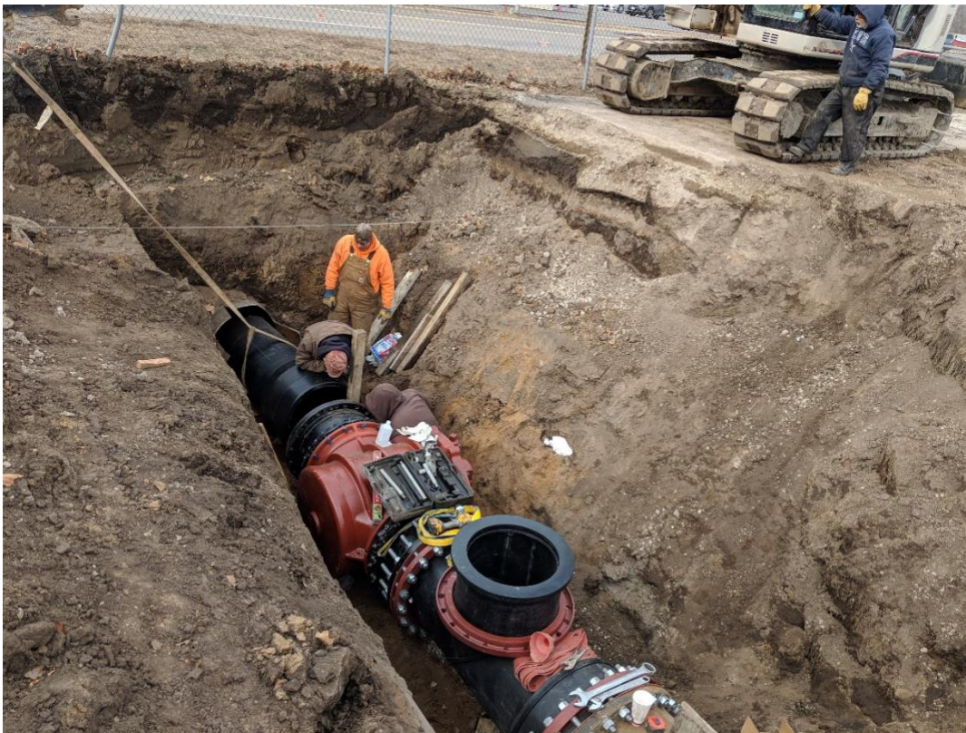
Musser Park connection and valve assembly for next phase 30" install to WPCP January 31, 2018
