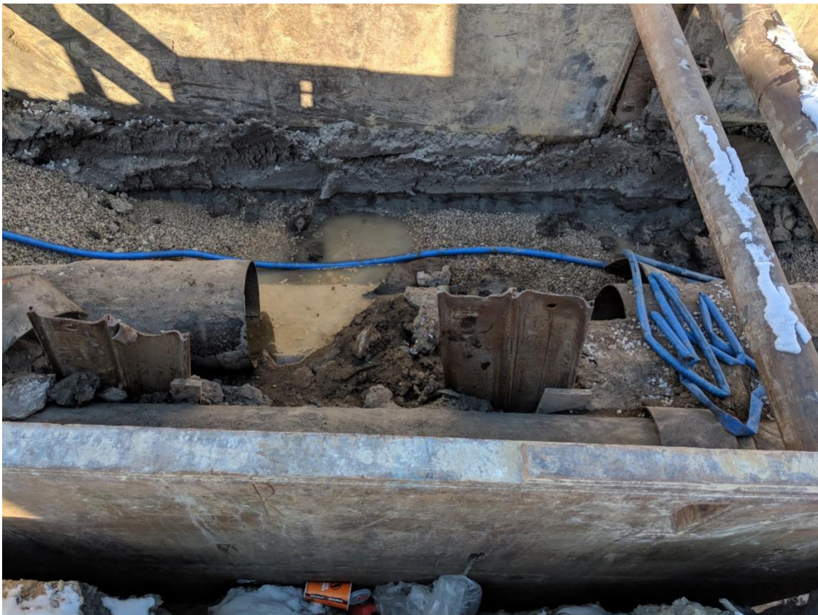
The pipe was cut and moved away from the 36" WPCP effluent line running parallel January 16, 2018
