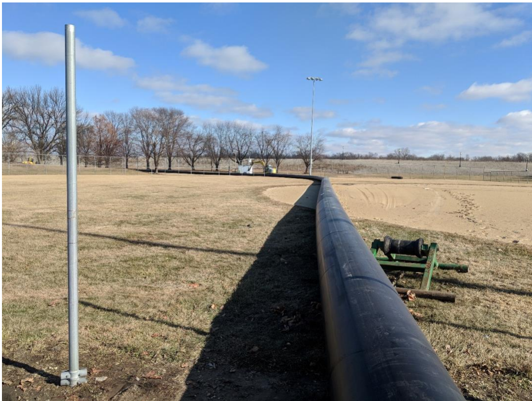
Fused 26" pipe laid out in Musser Park ready to be pulled through existing 30" January 27, 2018.
