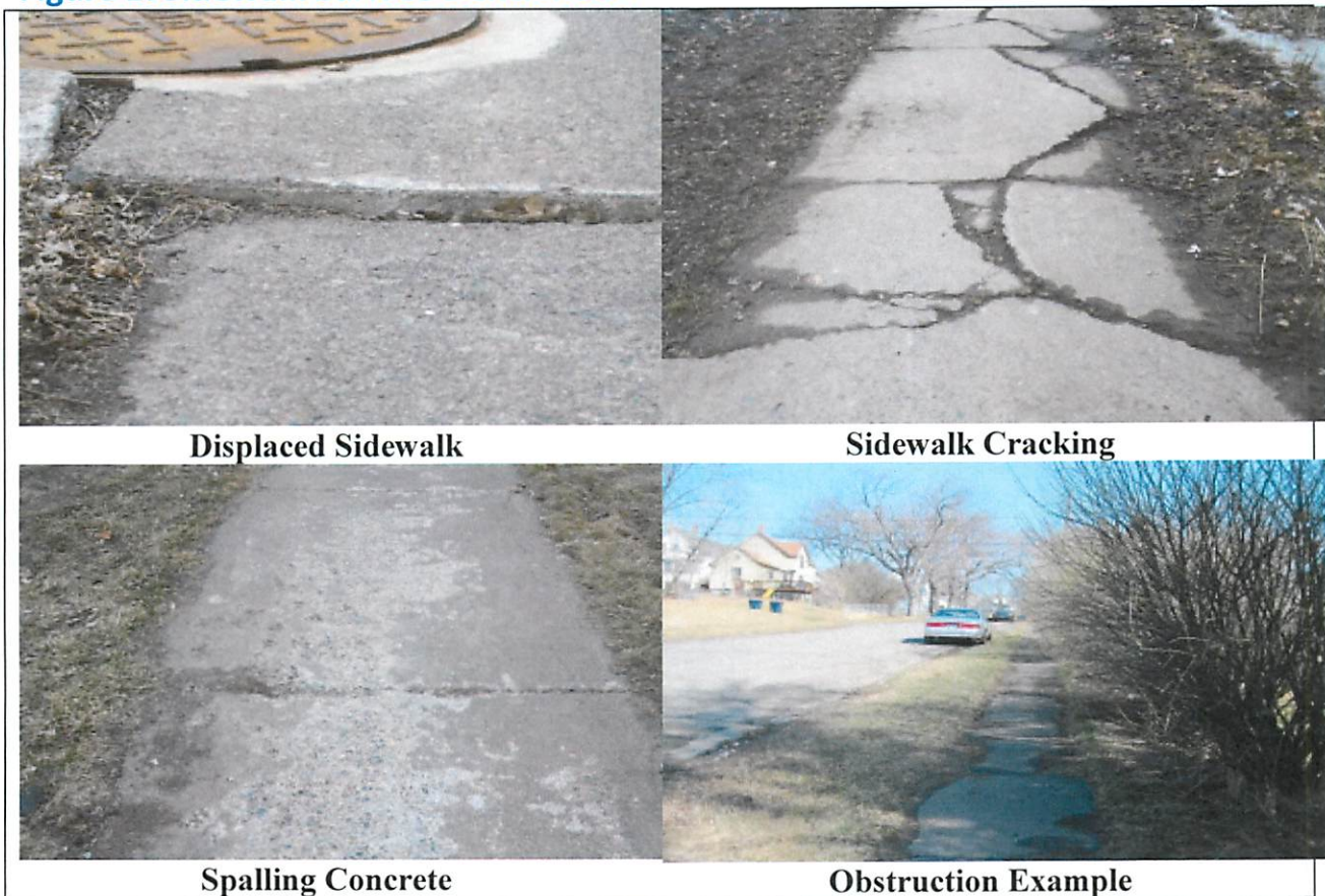
Figure 1: Sidewalk Surface Deficiencies 5
