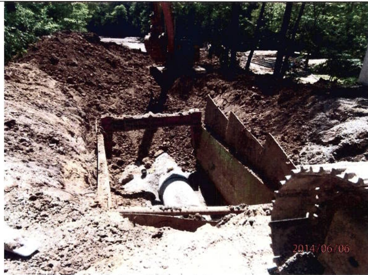
Upper end of ravine fill - 10" sanitary sewer pipe
