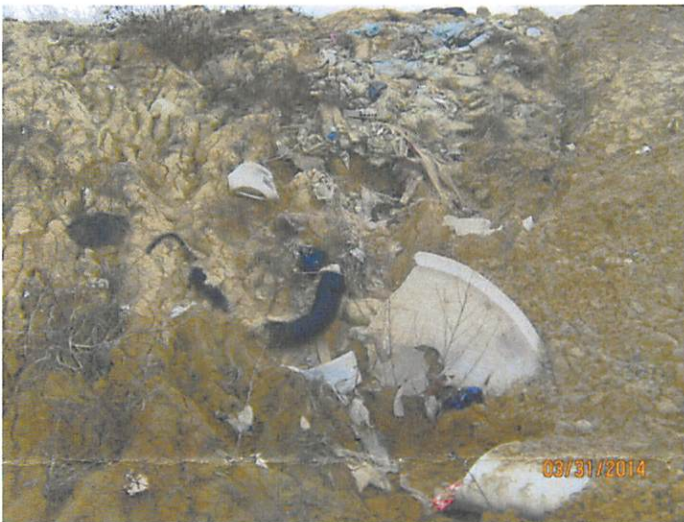
Photo 3: Photo taken 3/31/14, another example of exposed waste protruding through the cover soil.
