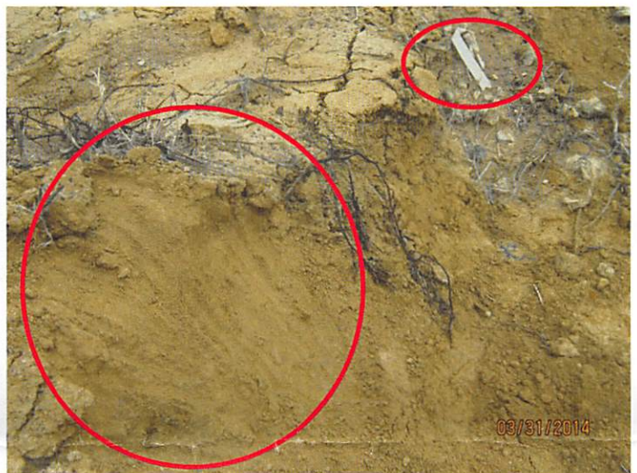
Photo 4: Photo taken 3/31/14, appears as though finger marks are in the dirt (inside the large red circle), indicating the amount of effort expended at covering the FML.
