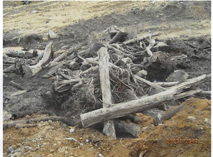
Photo 2: Photo taken 3/31/14, logs have clearly not been removed from the fill area, and it does not appear as though removal is scheduled, as cover soil has been dumped on some, and around the logs in photo #2.
