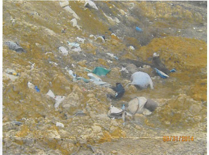
Photo 2: Photo taken 3/31/14, photo shows uncovered solid waste. Proper compaction is also questionable, on such a steep side slope.
