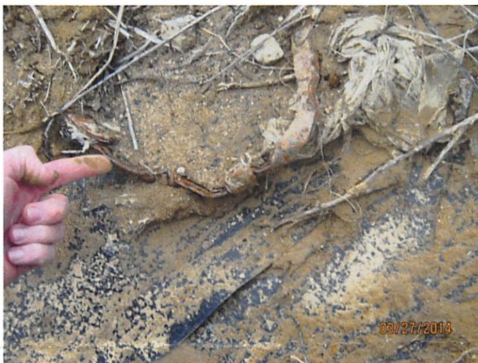
Photo 3: Photo taken 3/27/14, the red arrow in Photo #1 shows the same piece of metal as is shown in photo #3. It is unknown whether or not the piece of metal was removed prior to covering the FML (prior to Mr. Noll's announced visit).
